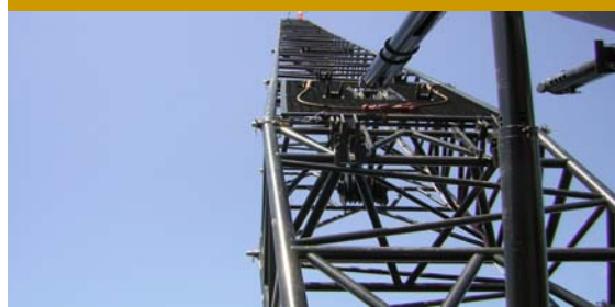
80 Ton Crawler Crane October 2007
